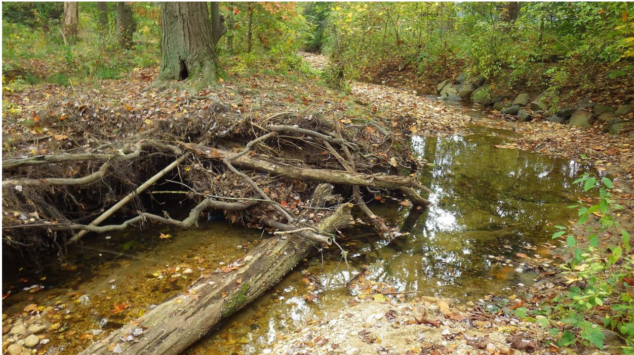
Fig. 2. Ten-year-old, failed NCD project along Strawberry Run in the City of Alexandria, Virginia that is naturally stabilizing itself with wood snags and log jams, which trap sediment and provide aquatic wildlife habitat. The selective boulder armoring in sections of this small order, upper headwater stream was minimal and largely successful (right background of photo). Photo by R.H. Simmons.
