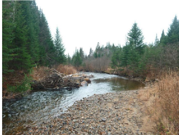
Figure 5. A meander developed around a marginal log jam constructed on an artificially straightened section of Nash Stream in Coös County, NH.
