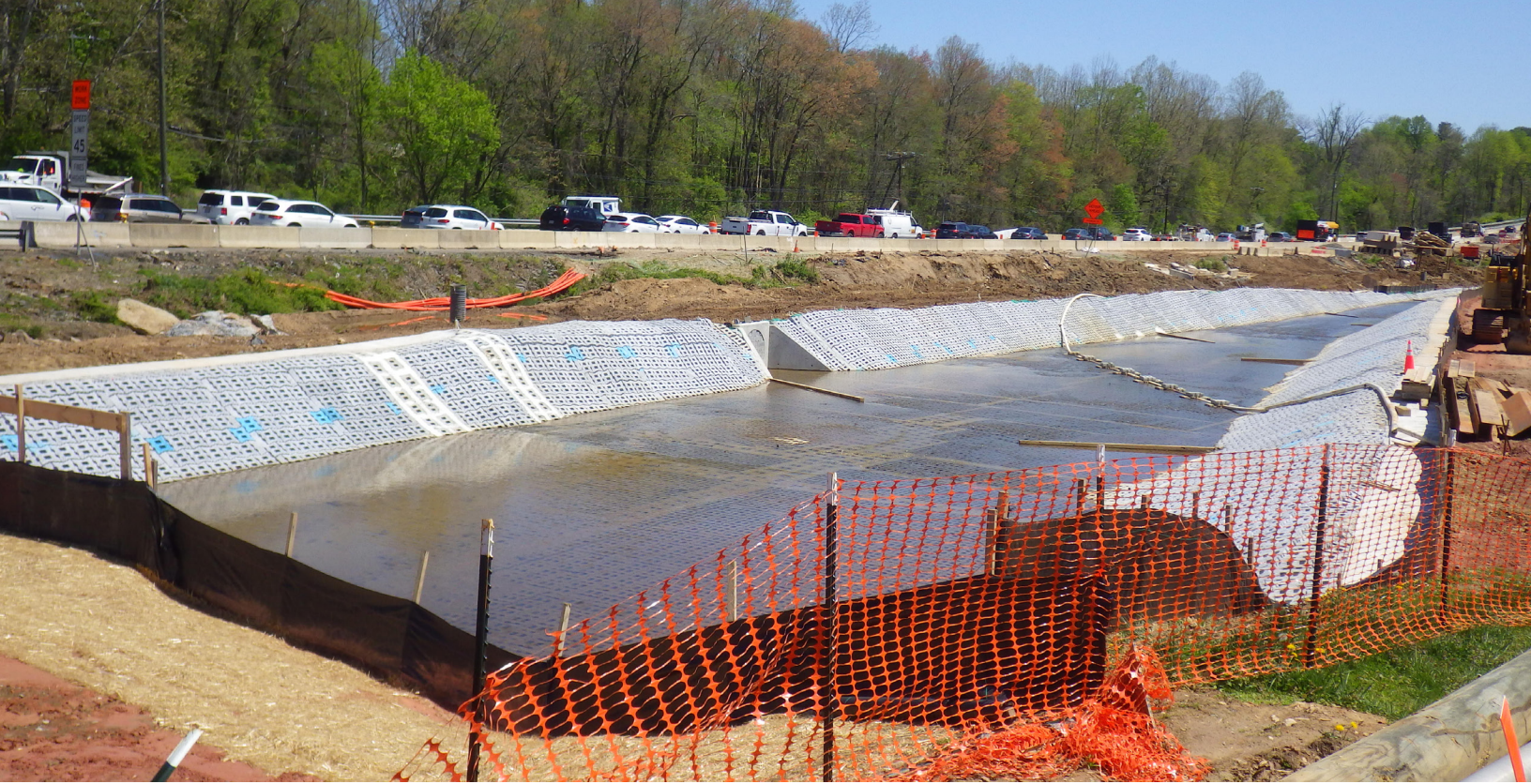
Fig. 4. A recently constructed massive drainage channel replacing a section of 1960s-relocated Colvin Run in Fairfax County, Virginia. Leesburg Pike (Rt. 7), shown in photo center, is being doubly widened. A large Piedmont / Northern Coastal Plain Basic Seepage Swamp (USNVC: CEGLo06406) runs along the south side of the above channel outside of the right photo frame. Despite the denuded, degraded landscape, the concrete channel is the only way to confine and accommodate enormous quantities of stormwater runoff from the widened roadway and environs without transferring it to forested wetlands and stream valleys, especially with 72" culvert outfalls aimed at said wetlands (middle left of photo). Photo by R.H. Simmons.
